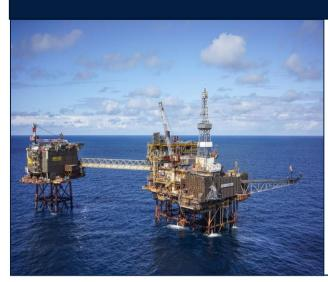
The Claymore platform, installed in 1976, is located 100 miles (161km) North East of Aberdeen. The complex contains two fixed steel bridge-linked platforms, the Claymore Production platform (CPP) and Claymore Accommodation Platform (CAP), connected by a 106m bridge. The CPP sits on a conventional eight-legged steel jacket, providing processing and drilling facilities. The CAP is much smaller and provides accommodation, utilities, and the helideck.
