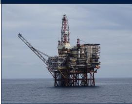
The Clyde platform, installed in 1986, is located 175 miles (280km) South East of Aberdeen. It is an eight-leg fixed steel jacket and module support frame, with drilling, production, accommodation and associated facilities.
