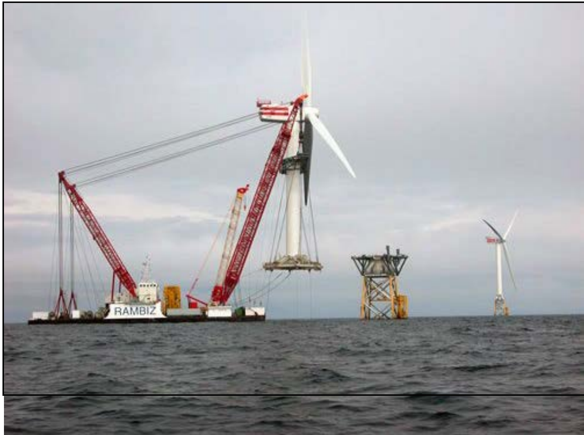
Figure 2.11 – Crane Barge Installing the Second Beatrice Wind Farm Demonstrator Turbine
